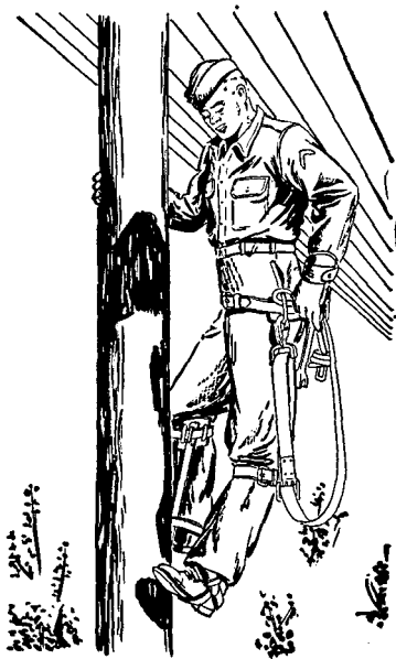
Figure 48. Unhooking safety strap.
