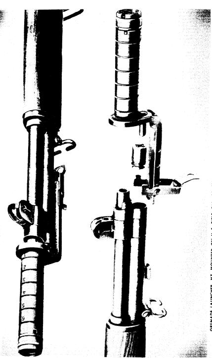
GRENADE LAUNCHER, M7, MOUNTED ON U. S. RIFLE, CAL. .30, M1, AND (BELOW) LAUNCHER DETACHED SHOWING VALVE SCREW TO REPLACE GAS-CYLINDER LOCK SCREW
