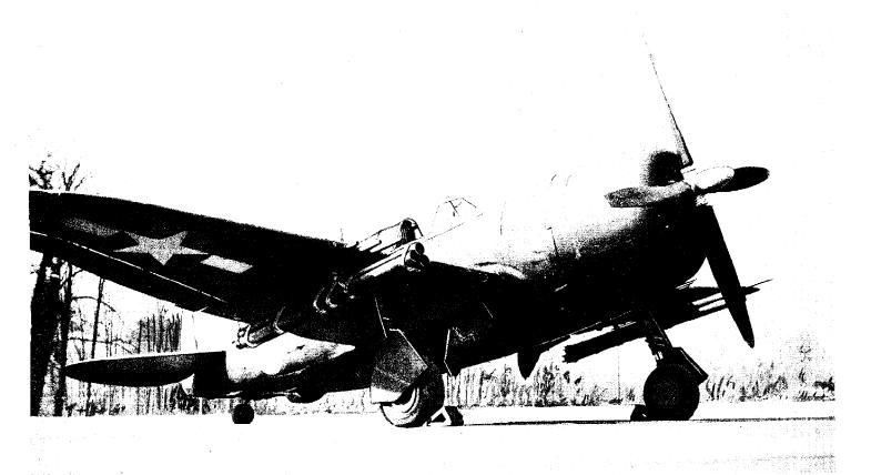
4.5 INCH 3-TUBE AIRCRAFT ROCKET LAUNCHER, M15, MOUNTED ON P-47 PURSUIT PLANE
