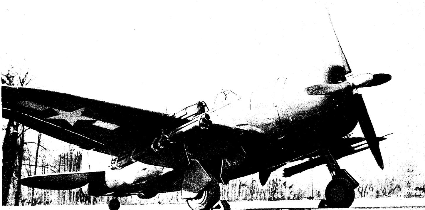
4.5 INCH 3-TUBE AIRCRAFT ROCKET LAUNCHER, M15, MOUNTED ON P-47 PURSUIT PLANE
